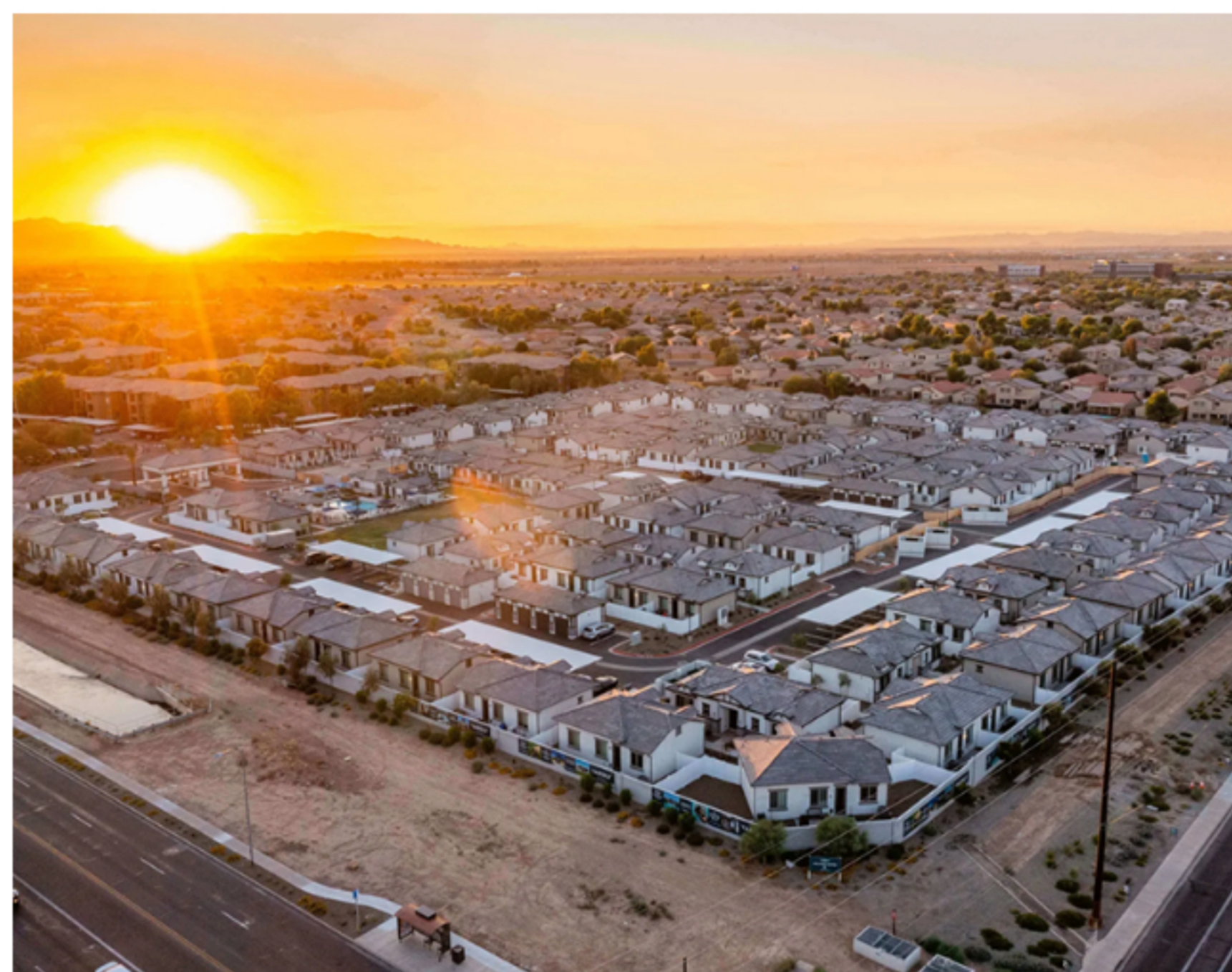
Yardly McDowell, a 167-unit, BTR property located in the West Valley of Phoenix, Ariz. Image courtesy of Tower 16 Capital Partners
